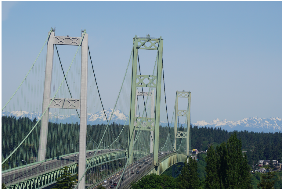
Figure 4.4.11 The Tacoma Narrows Bridge (2017)
