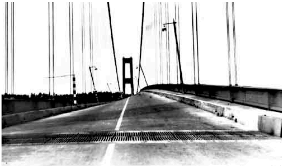
Figure 4.4.10 The Tacoma Narrows Bridge
