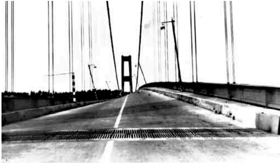
Figure 4.5.5 The Tacoma Narrows Bridge
